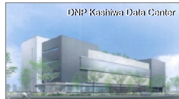
Total floor space 10,580m 2 ( 850 racks )
